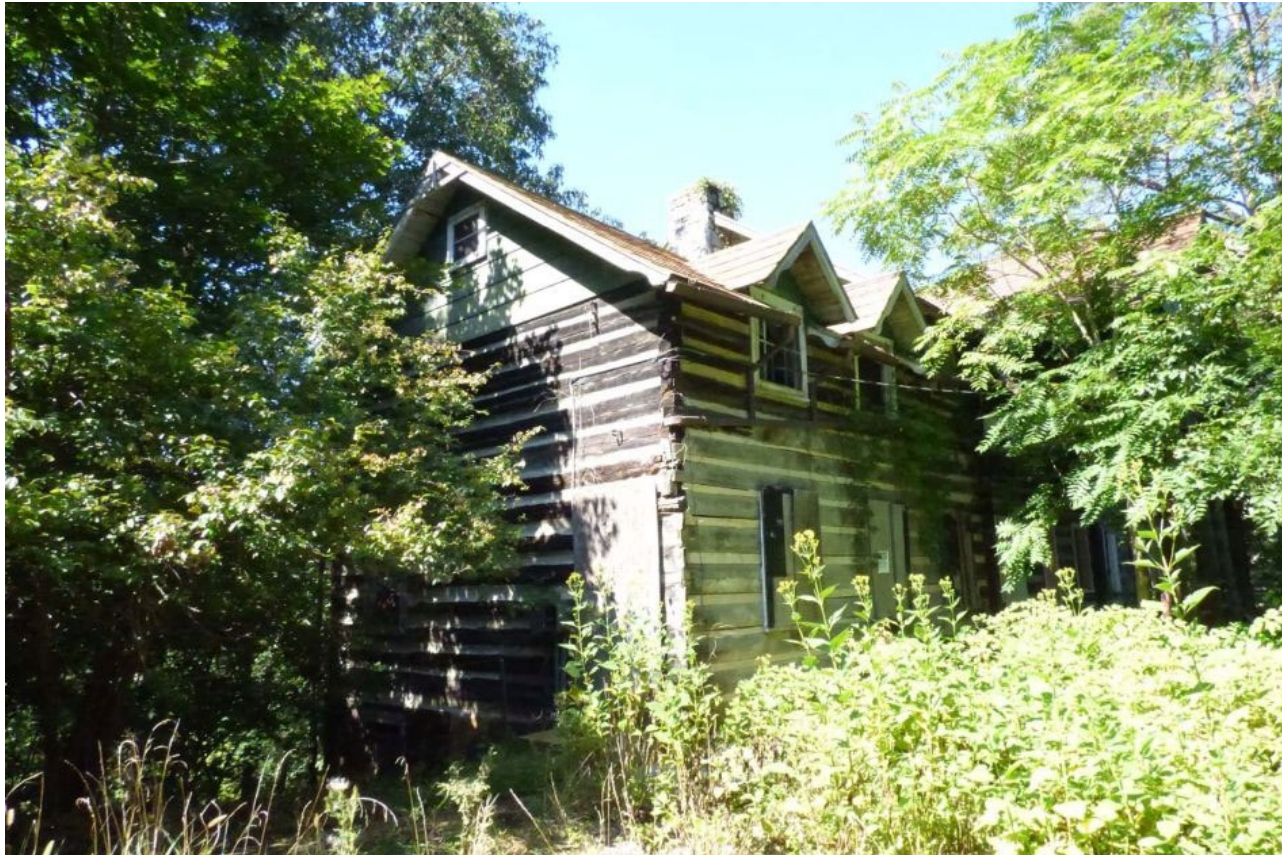
Image 5. One of the Camp Lupton Cabins that were on the Seven Bends State Park property. Although none of the original camp buildings exist on the site, the site is still considered historic by DHR. Photo By Department of Historic Resources, https://vcris.dhr.virginia.gov/VCRIS/Mapviewer/
